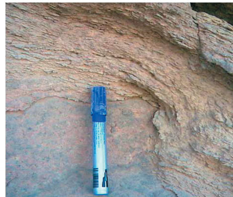
Fig. 4: Close up view showing exfoliation in younger granites, looking NE
